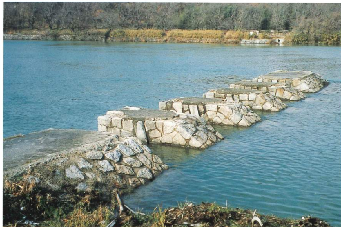
69 Weir of the old head works of the Meiji-Yosui irrigation channel (presently Yahagi River in Toyota City), built by Choshichi Hattori in 1909 and completed with artificial stone techniques.
