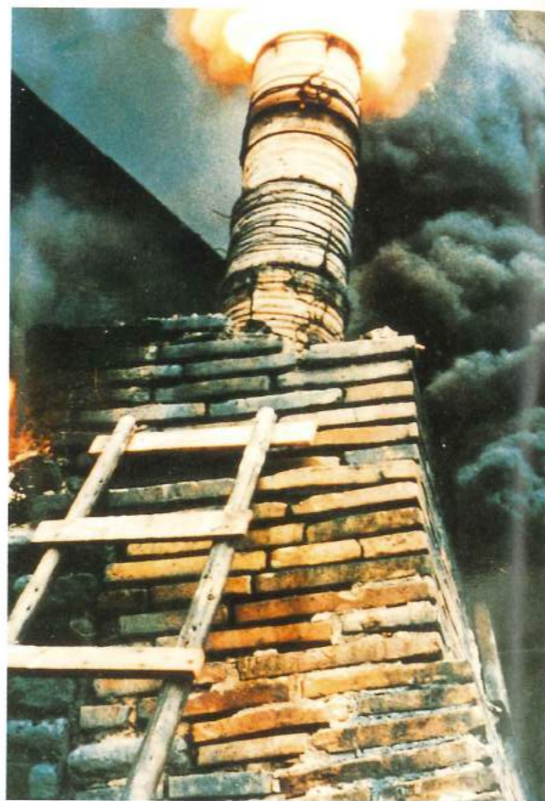
19 Accessory chimney of Hora Kiln, in Seto City, in use from 1949 to 1979.
