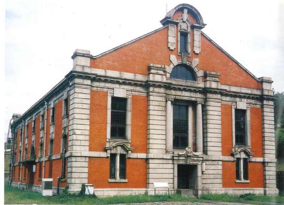
7 The first pump house of the Nabeyaueno Cleaning Bed, built in 1914. It was Nagoya's first water purification facility.
