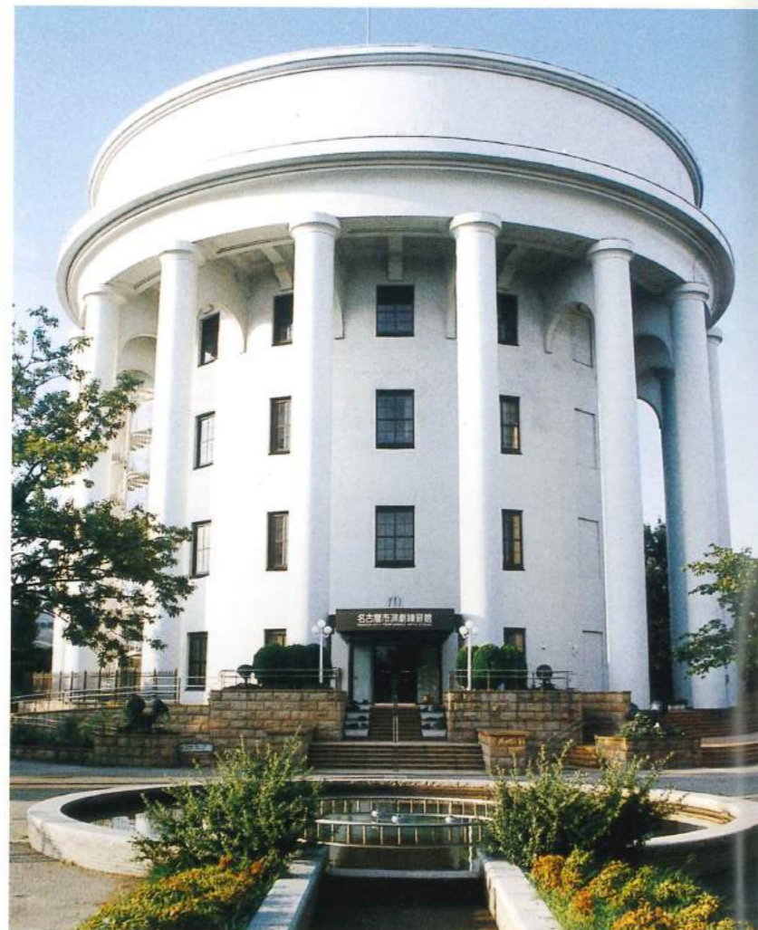
The Inabaji Water Tower, built in 1937, a cylindrical structure with a diameter of 33 meters and a height of 29.47 meters, and supported by sixteen cylindrical pillars.
