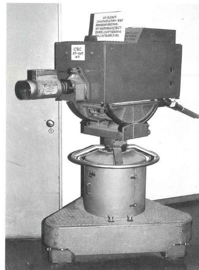
54 The first color television camera made entirely from transistors, built in 1962 by Chubu Nippon Broadcasting Company.
