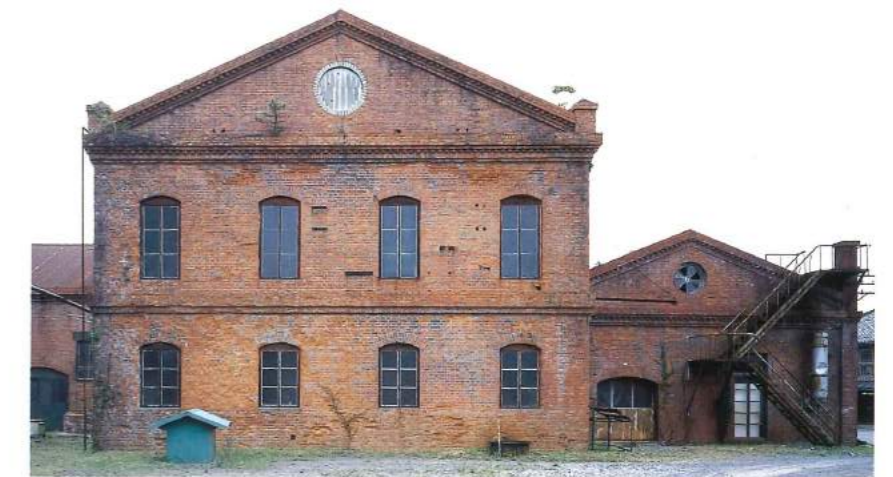
30 The Kitakawa Manufacturing Company building, situated near the Ooi River, is a brick structure that was built between 1898 and 1935 which was used for dry distillation of wood.
