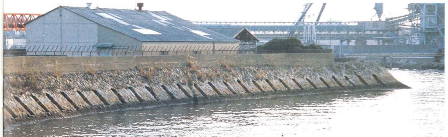
67 Designated as an Important Cultural Asset in 1996, the old Yokkaichi Port's breakwater was constructed in 1894 by Choshichi Hattori and is characterized by small holes from which water is allowed to spout.
