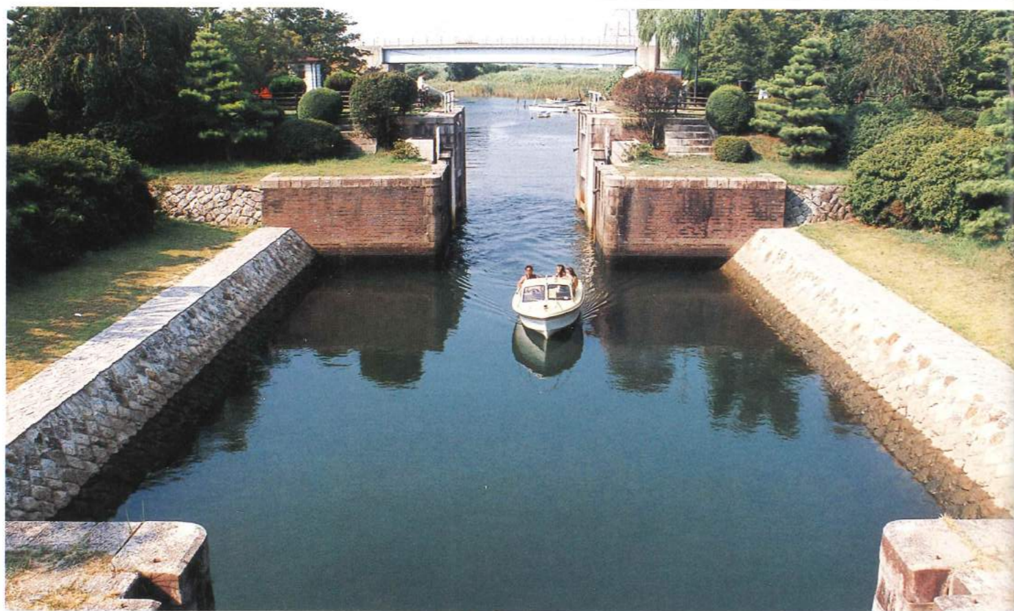
79 Sendohira Lock, built in 1902, allows the passage of 100 to 500 fishing ships and leisure boats per year.
