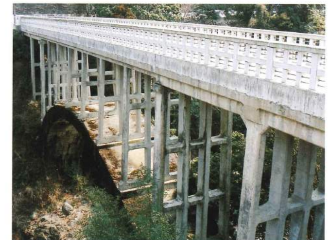
77 Tsuge Bridge is an open-arch bridge made of reinforced concrete and has long pillars connecting the bridge and the arch portions. Built in 1918, it is a beautifully designed bridge.
