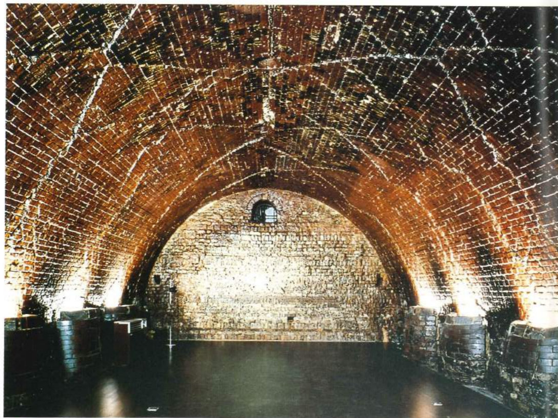
22 Interior of the limekiln in Kiln Plaza and Museum, built in 1921. With a frontage of 5.5 m, depth of 11 m, and height of 3.4 m, this kiln produced earthen pipes for 50 years.
