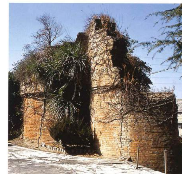
24 Remains of the Tokkurigama, in use from 1889 to 1924 to make cement, seen on the grounds of Mikawa Cement Company.
