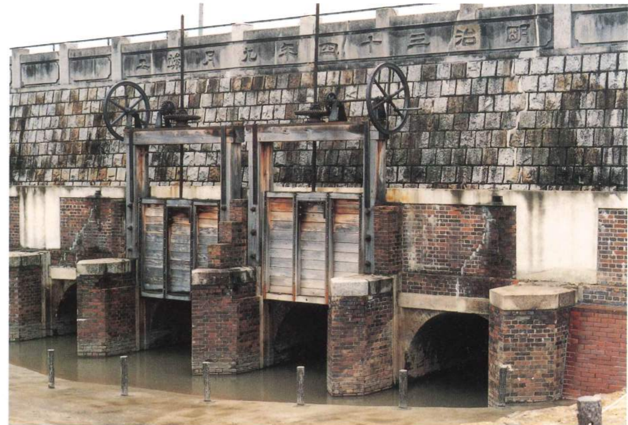
80 The upstream side of the Tatsuta-Waju Draingate, built in 1901.
