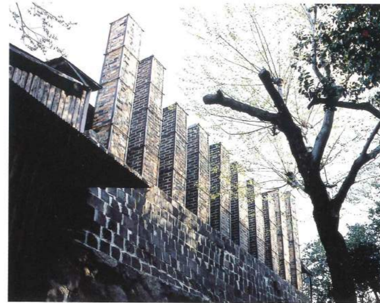
26 Cluster of 10 chimneys at Toueigama, a Noborigama built in 1887 in Tokoname and now designated as an Important Cultural Asset.
