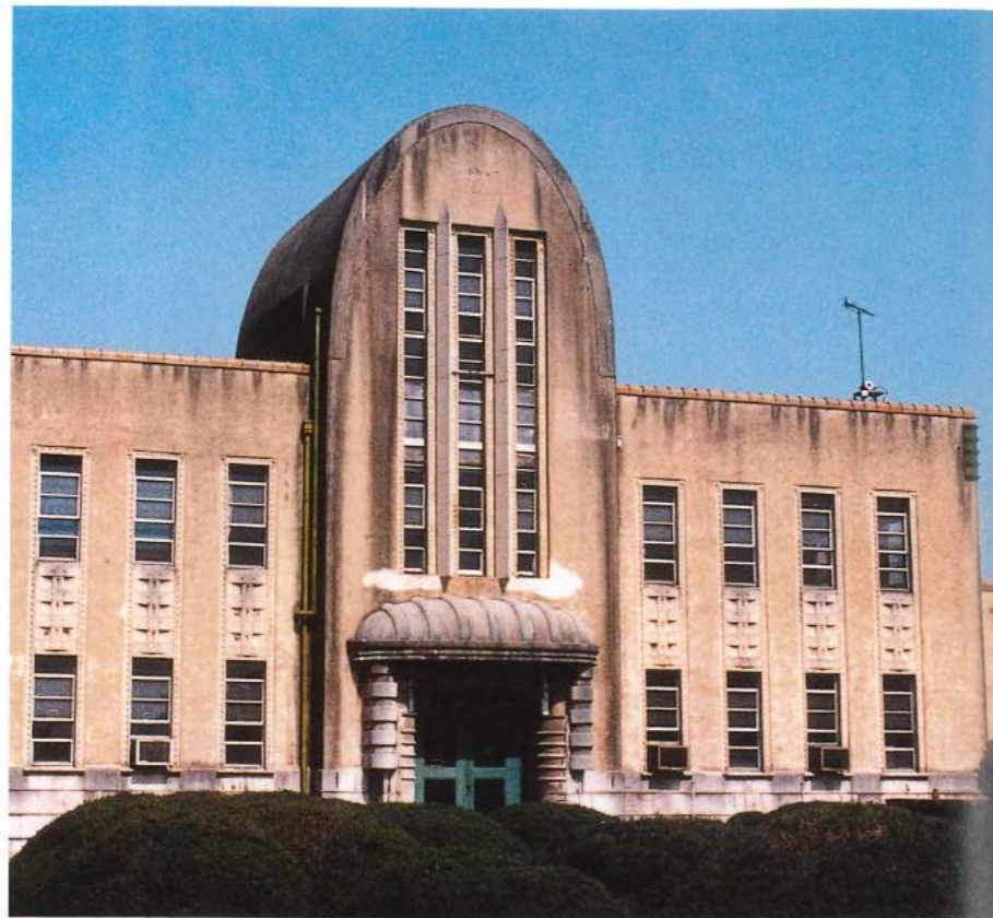
50 Yosami Radio Transmitting Station, where the first radio communication between Japan and Europe took place in 1929.
