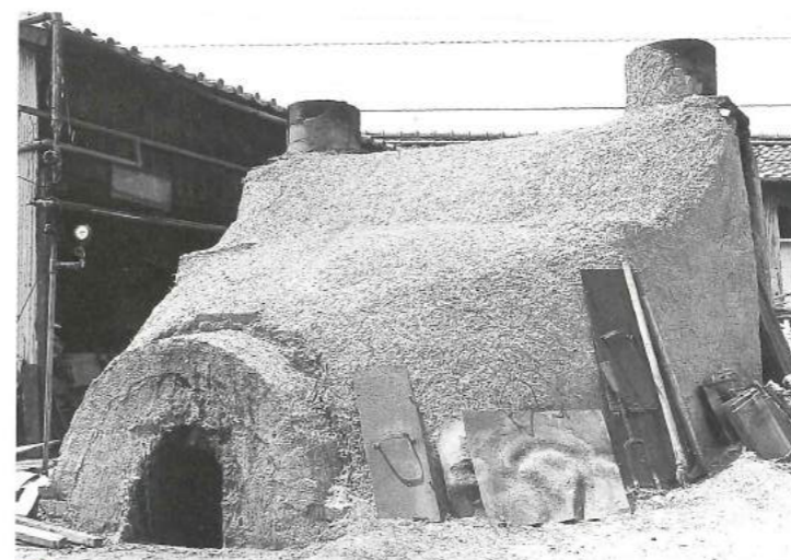
23 The Darumagama in Takahama City, built in 1923. For 70 years it produced the roofing tiles known as Sanshu-Gawara. Designated as a Traditional Cultural Asset in 1999.
