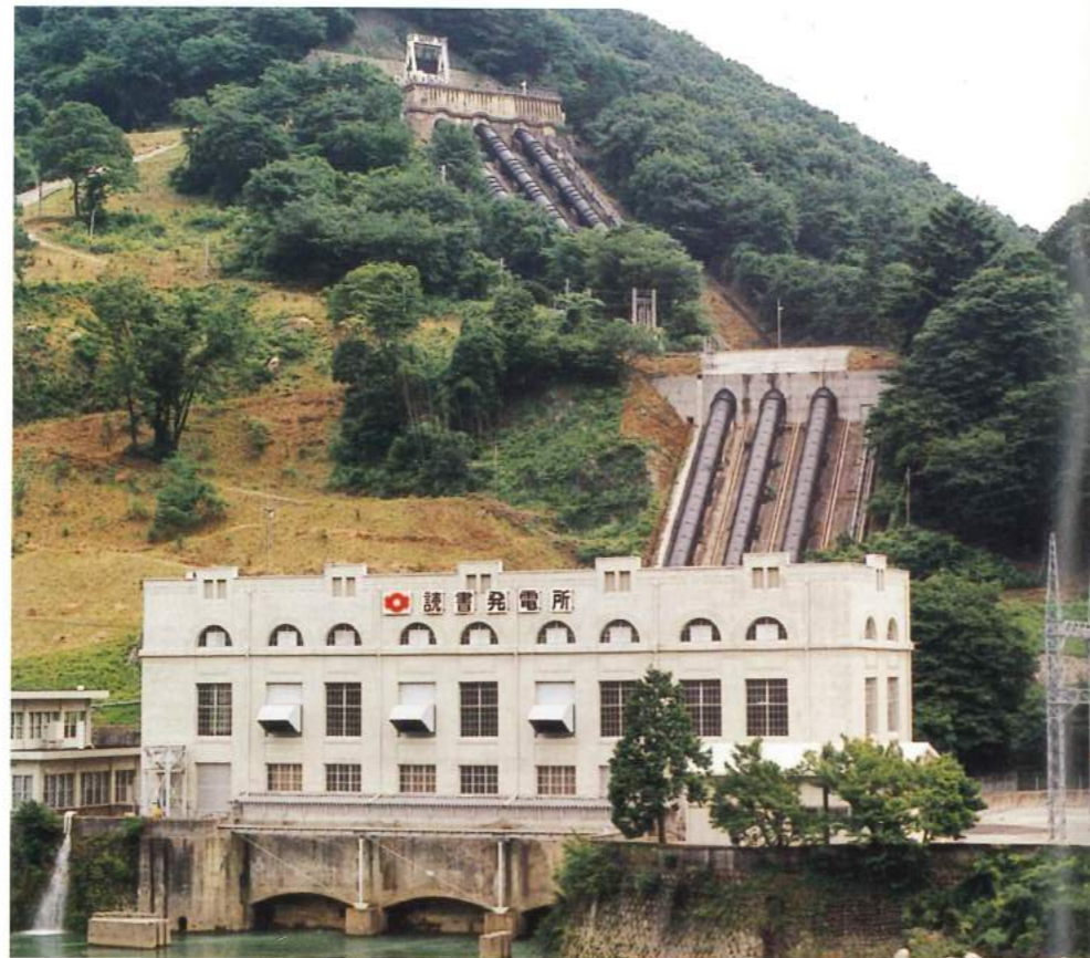
31 The Yomikaki Power Station, built in 1923, has an output of 40,700 kw and utilizes water from the Kiso River. It has been designated as an Important Cultural Property.
