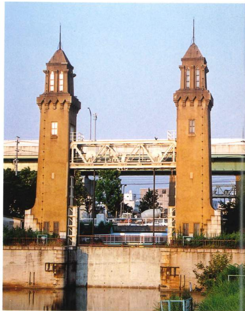
92 The Matsushige Gateway was completed in 1932 to connect the Nakagawa Canal and the river Horikawa. Since the water level in Horikawa is higher than that in the Nakagawa Canal, ships were passed through the gateway while adjustments in water level were being conducted. Two of the towers support the winding apparatus that is used to open and close the 40-ton doors to the gateway. At one time, the gateway passed 90,000 ships per year, but with the increase in truck transportation, it was forced to cease operations in 1968.
