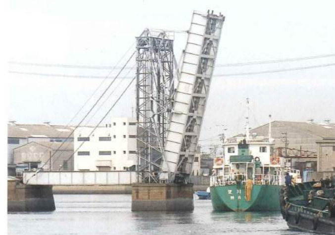
74 The old Yokkaichi Port Railway Bridge, built in 1931, is the oldest working drawbridge in Japan. The 26.6-meter movable portion is drawn up through a system of ropes and pulleys over a period of one minute 20 seconds.
