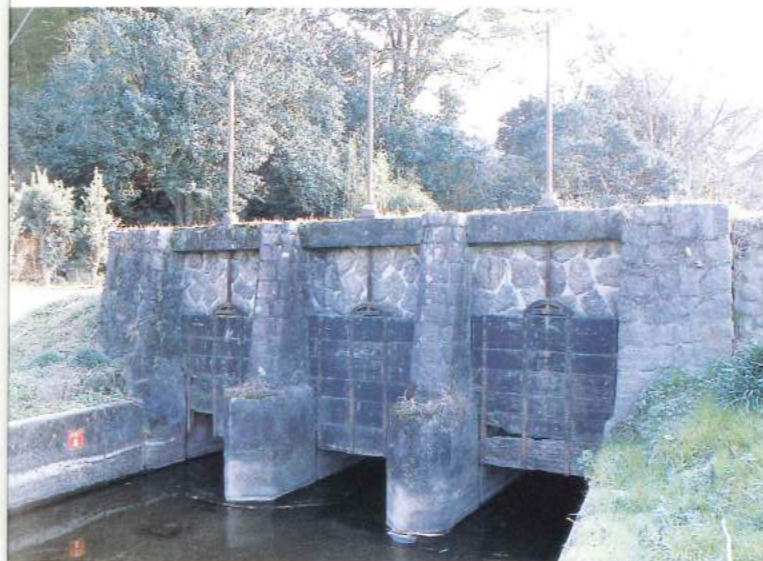
70 The No. 5 Watergate of Muro Sluiceway, made from artificial stone in 1894.
