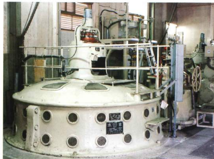
33 Generator house of the Nagashino Power Station, with Japan's first vertical-axis type generator, 1912. The generator could be used in areas with very little altitude difference, and it soon spread nationwide.
