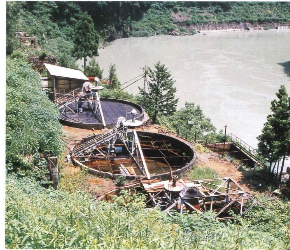
64 The Dorr thickener used at Kune Mine, which stirred and caused sedimentation of the copper-ore pulp to alter its solid density.
