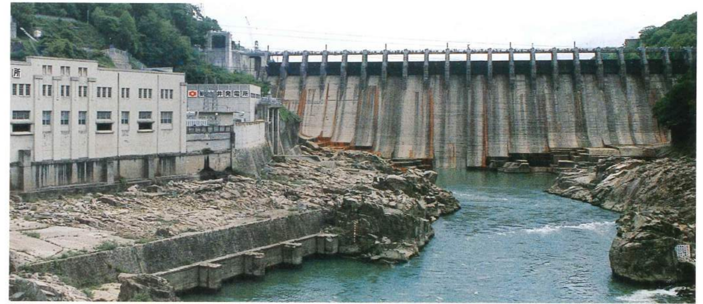
32 The Ooi Power Station, with an output of 42,900kw, and the Ooi Dam, with a height of 53 m, were the largest of their kind when they were built in 1924. Traditional log-rolling down the river was replaced by log transport using the Forest Railways.
