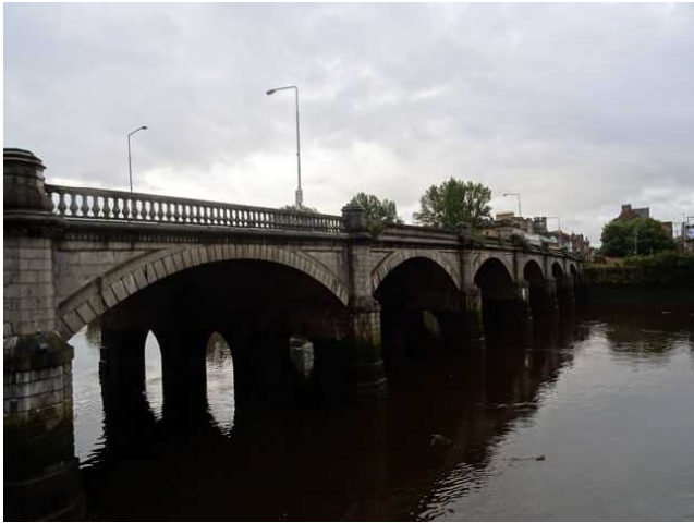
[写真10] The Glasgow Bridge
